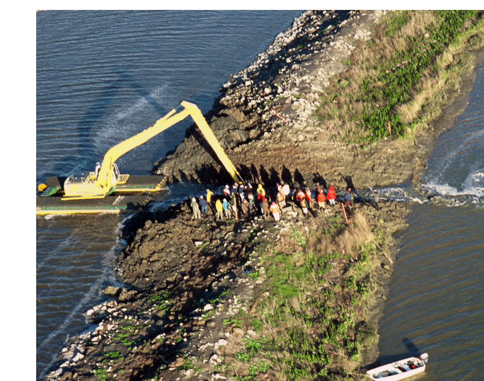
Excavator Levee Breach, Alviso Island Ponds Marc Bittner, 2007
